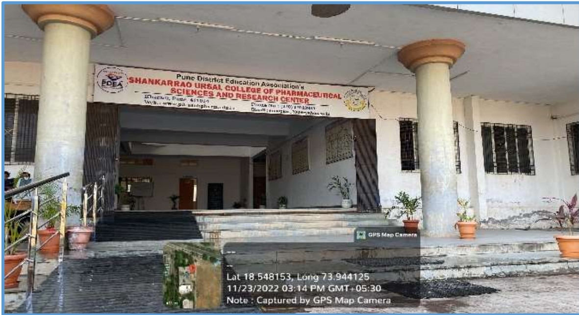
Ramp at college Entrance
