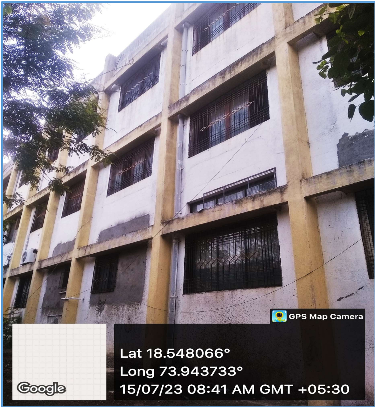
Rain Water Harvesting System
